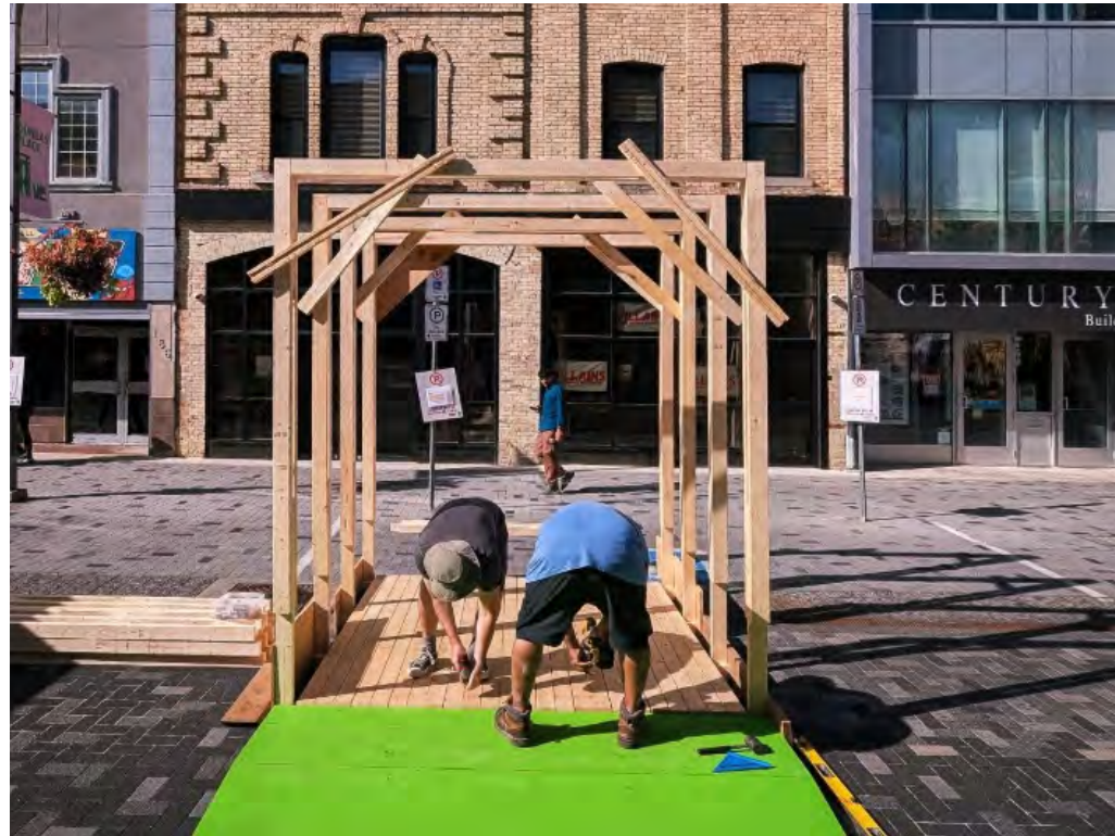
Assembly of the LSA installation at Nuit Blanche London.
